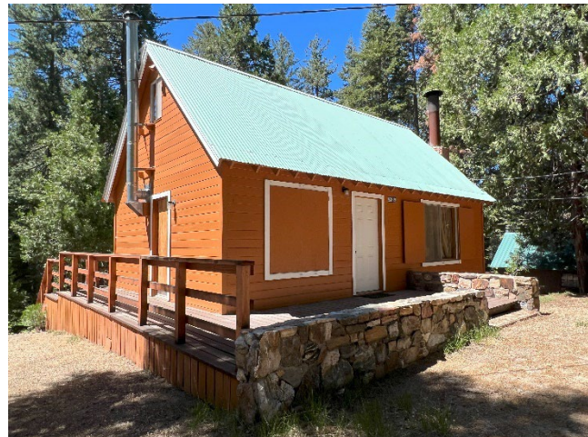
Building No. 92, 83819 Laurel Lane (Photo No. 0004).
