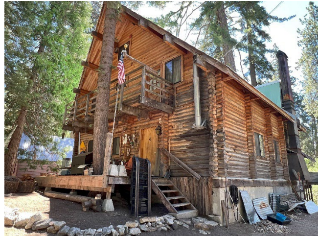
Building No. 94, 83827 Laurel Lane (Photo No. 0006).
