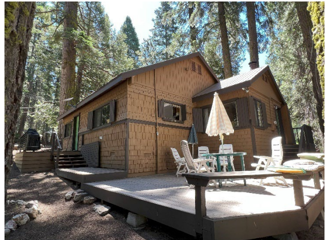
Building No. 105, 83793 Lily Lane (Photo No. 0008).
