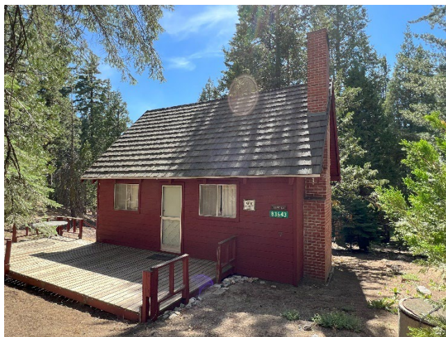
Building No. 134, 83643 Park Road (Photo No. 0009).
