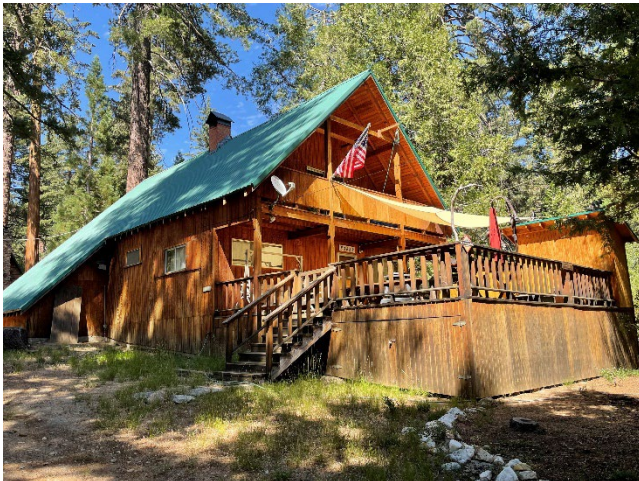
Building No. 101, 83852 Lilac Lane (Photo No. 0007).
