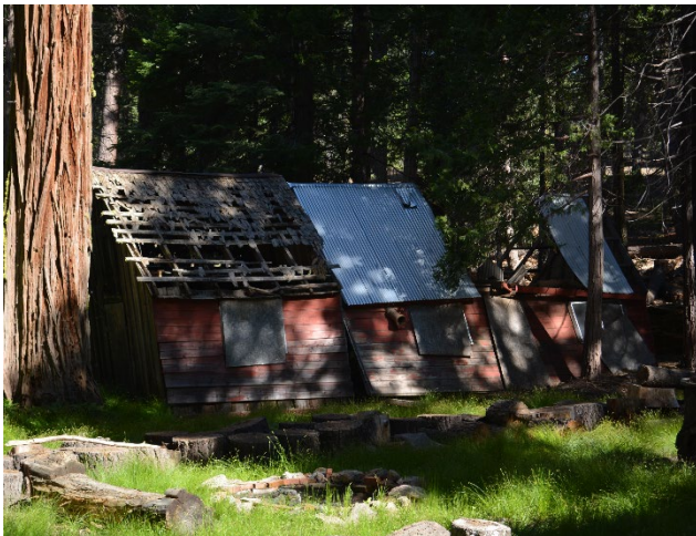
Building No. 29, 83792 Fern Lane (Photo No. 0017).
