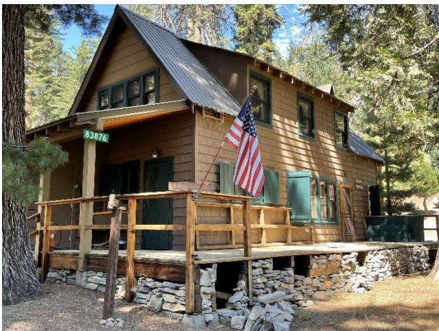
Building No. 103, 83876 Lilac Lane (Photo No. 0019).
