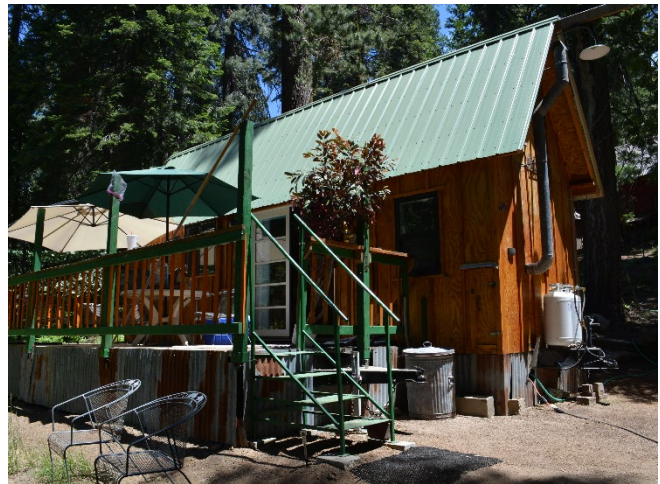
Building No. 213, 83649 Chinquapin Lane (Photo No. 0022).
