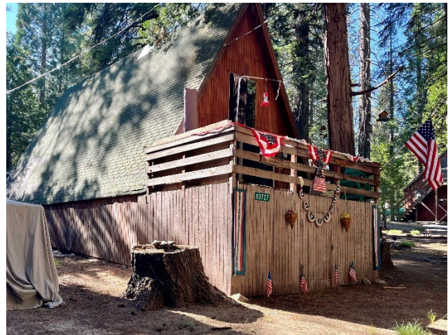
Building No. 18, 83727 Cedar Lane (Photo No. 0002).
