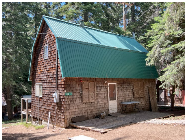
Building No. 154, 83643 President's Lane (Photo No. 0010).
