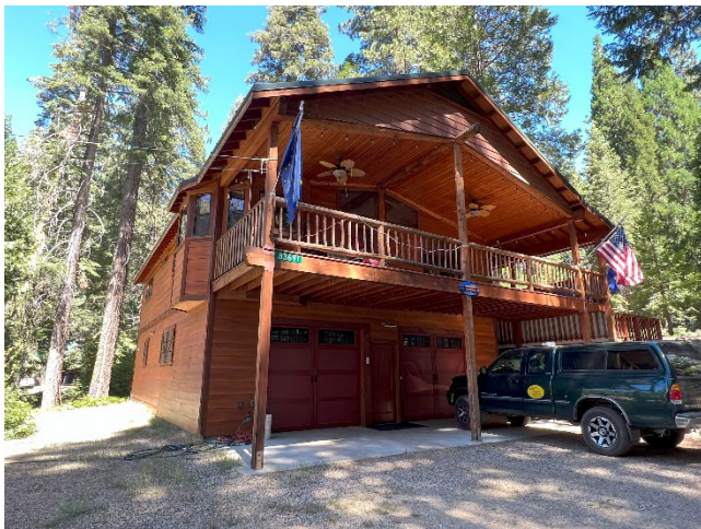
Building No. 212, 83691 Cedar Lane (Photo No. 0021).
