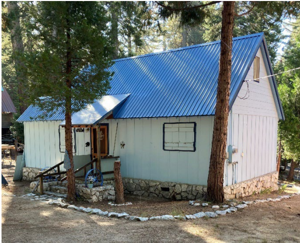
Building No. 93, 83823 Laurel Lane (Photo No. 0005).
