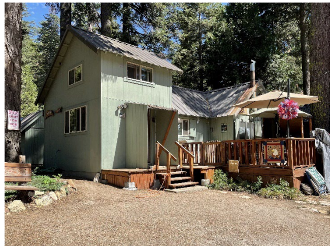
Building No. 97, 83815 Lilac Lane (Photo No. 0018).
